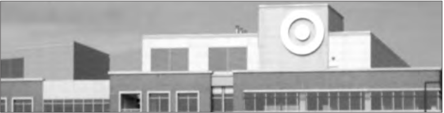
Target Northwest Campus Corporate Headquarters. Photo: Tracy Nordquist
